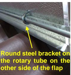
The scope of delivery includes two flaps up to a ridge of 30 m, which are already prepared with an eyelet for the traction rope, a round steel bracket for the locking device and the return spring (see picture on the right). If possible, the position for the locking technology should be chosen so that it is no more than 18 m away from the end of a locking section.
